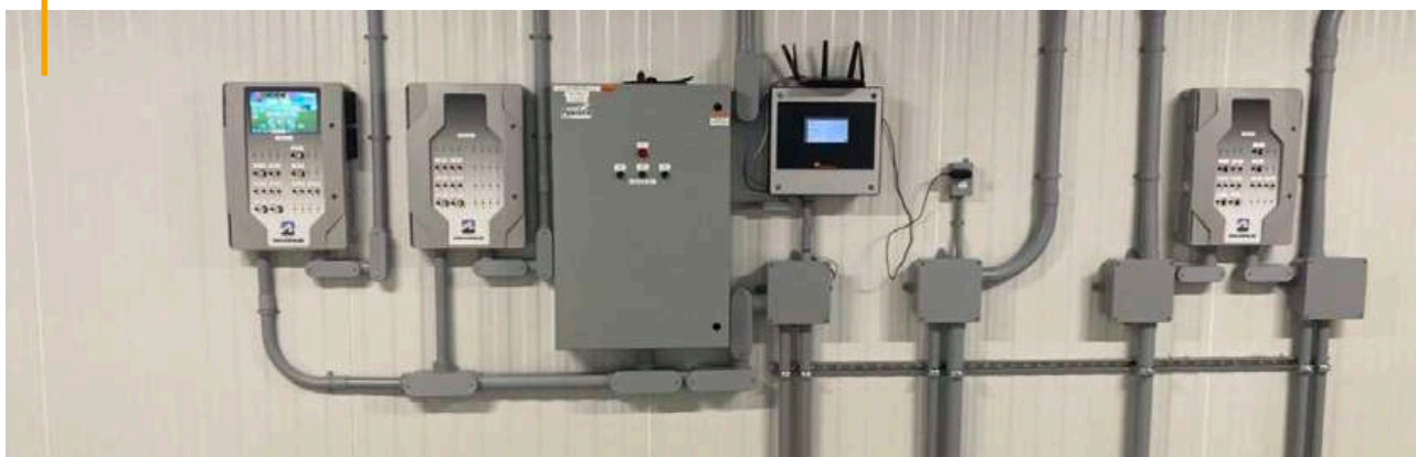
Ventilation controllers from a local supplier that are made in Canada are used in this new barn.
