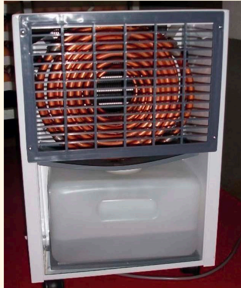
▼ Image 1. A dehumidifier installed in a pre-warming room, with its reservoir being filled with water previously present in the air as vapor. By collecting this water, Relative Humidity in the environment drops to a level where dew point will never be reached when eggs are brought in.
